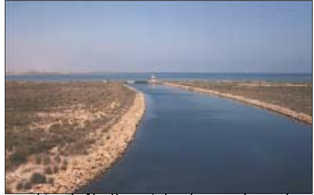
Fig. 7: Northern interchange channel.
