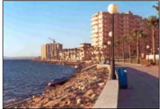
Fig. 11: The Mar Menor shore of La Manga with seawall construction.
