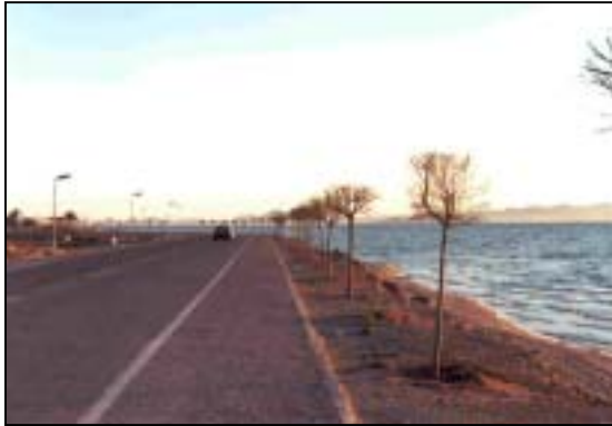
Fig. 10: Road built in the Mar Menor shore of La Manga.
